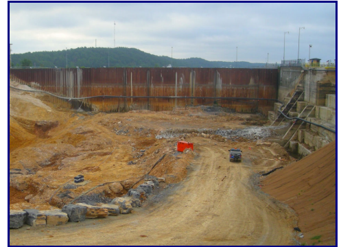
Excavation for new lock construction at Kentucky Lock
