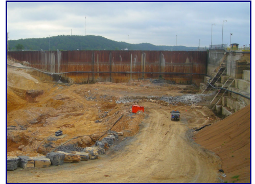
Excavation for new lock construction at Kentucky Lock
