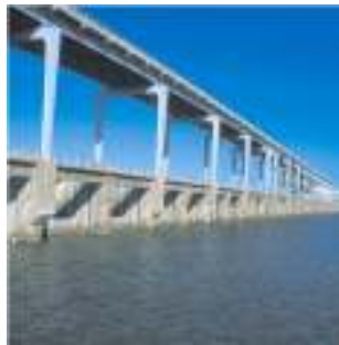
Flood damage reduction
