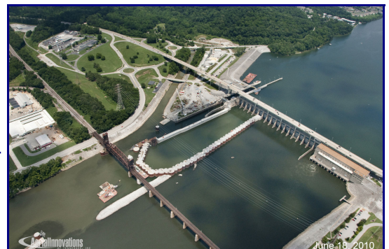
Cofferdam at the Chickamauga Lock Replacement Project on the Tennessee River
