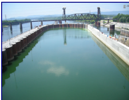
Completed Cofferdam at the Chickamauga Lock Project Site that will be pumped dry in the coming weeks. At that time construction is scheduled to be suspended for what could be as much as a decade without a resolution of the insolvency of the IWTF.
